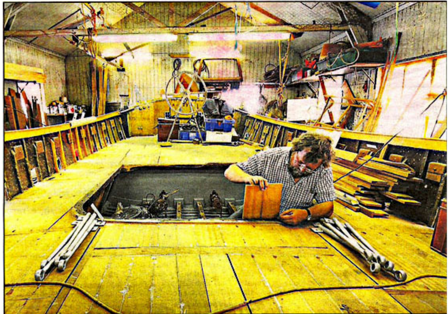
RENOVATION WORK: George Hewitt, busy restoring the Robert Lindsay.
